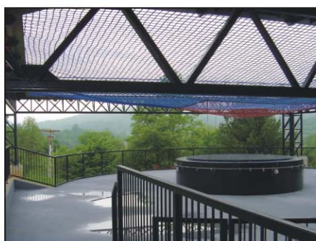
The tunnel opening from below the net.
