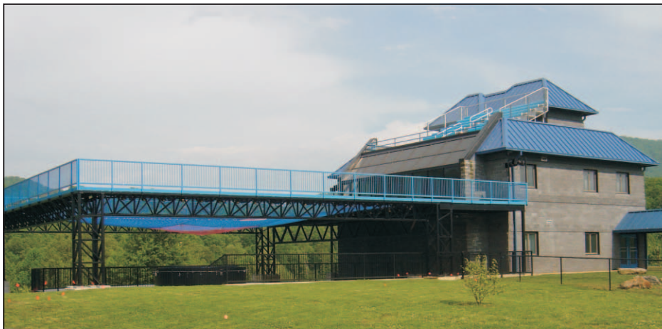
The wind tunnel facility at Waynesville. The flying area is on the left. The top of the tunnel outlet is below the deck.
