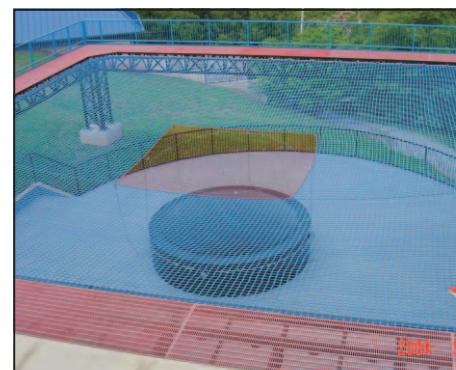
The tunnel outlet sits below the safety net.
